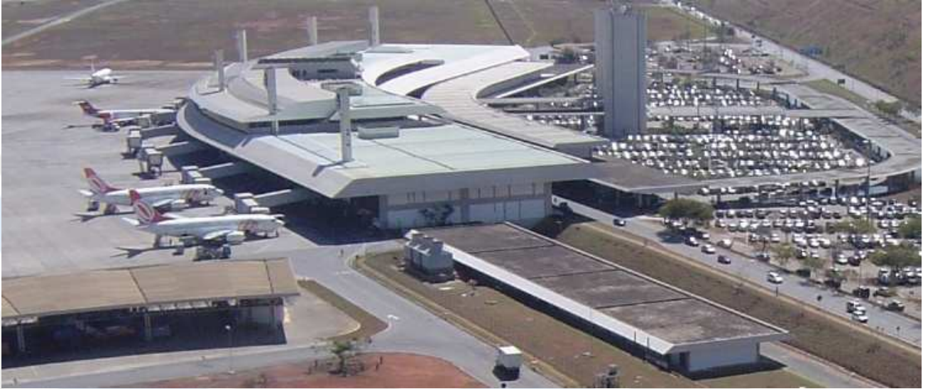
Figure 6 - Partial View of the Tancredo Neves International Airport
